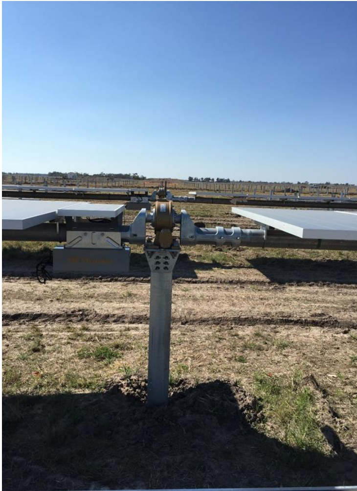
Plate 1: Indicative Single Axis Tracking
